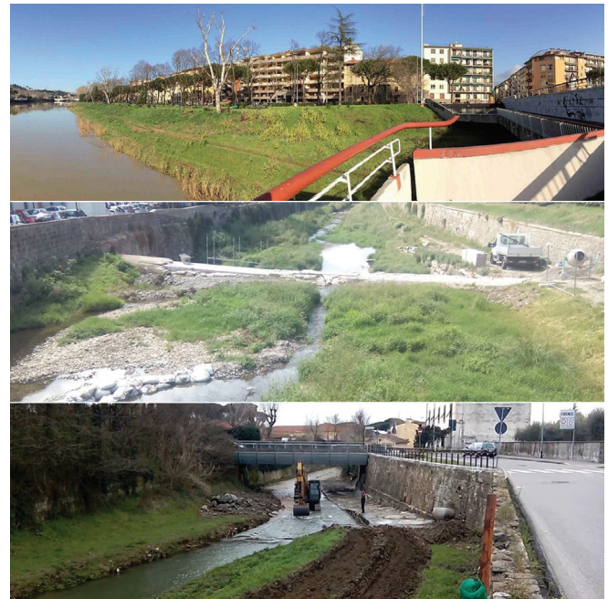
Figure 2. From above: Arno river and its surroundings areas, Mugnone river and Terzolle river during some riverbed arrangement work of 2017 (source: Own archive).
