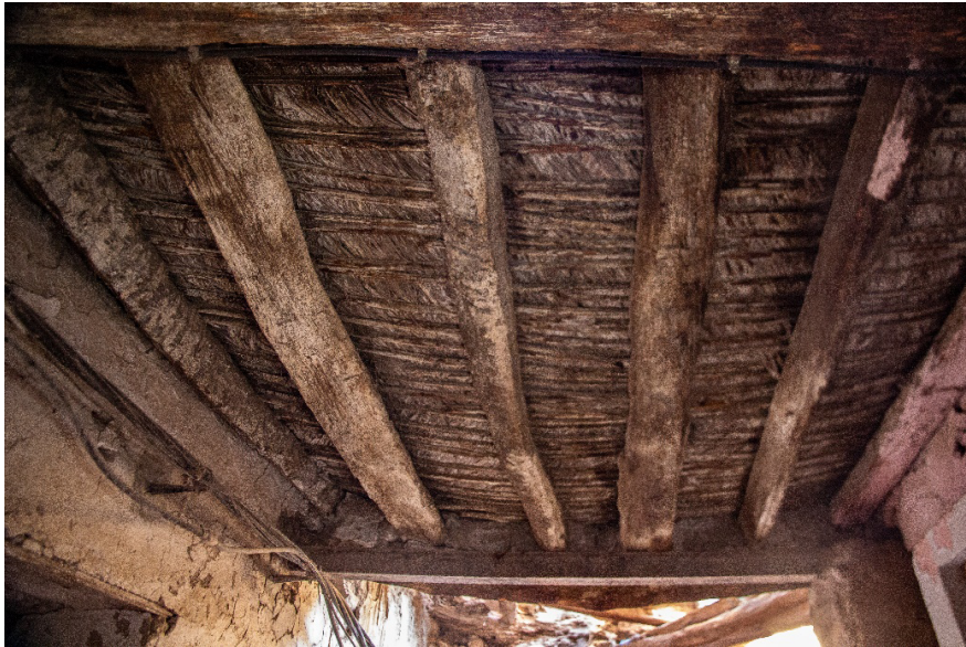
Image 2. Beams made of local materials (source: Authors', 2020).
