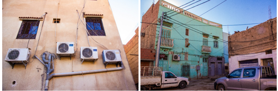
Image 9. Use of air conditioners (source: Authors' 2020).
